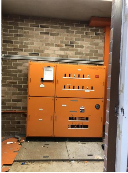
Figure 4: Existing main switchboard at APS (BR001)
